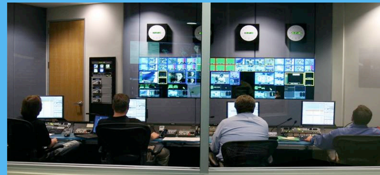
MediaFLO Network Operations Center (NOC), San Diego, CA
